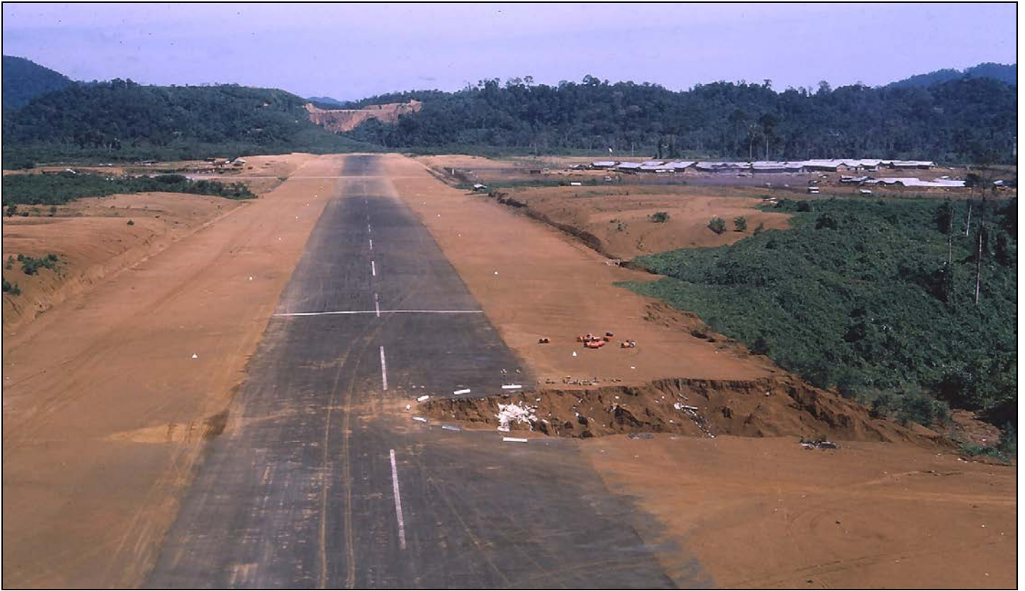
Wash-away at Kham Duc. Note ridge on approach bulldozed away to enable use by C-123s.
