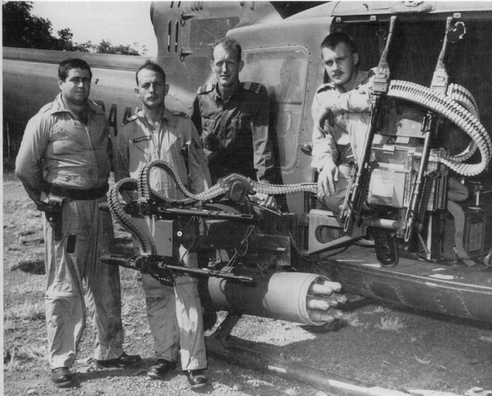
The first RAAF gunship, dubbed 'Ned Kelly', showing the trial armament system fitted to UH-1B A2-1025 in March 1968. Pictured with the aircraft are members of the project team (from left): Sergeant E.E. Moore, Flight Lieutenant R.C. Thompson, Squadron Leader J.H. Cox. At right is armament fitter, Leading Aircraftman E.G. Maxwell. (DEPAIR FILE 417/5/48[1], DD: AWM P01942.002)
