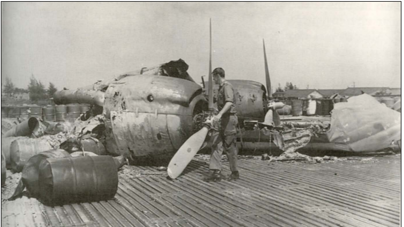
All that remains of Caribou A4-193 which was completely destroyed by enemy mortar fire at That Son in March 1970. The aircraft was carrying drums of helicopter fuel and the subsequent fire was so intense all that was left were the engines. The crew was forced to hurriedly abandon the aircraft and were lucky to escape without serious injury.
